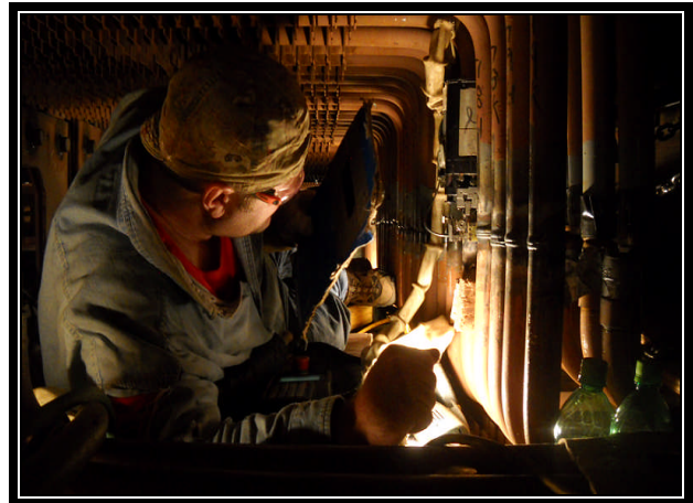
First Time Quality Production Welding
