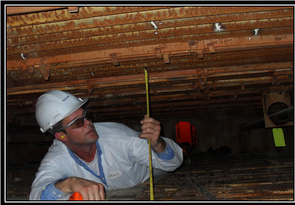
Restricted Access in the Economizer Section
